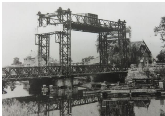
Class 70 Bascule Bailey Bridge being raised
