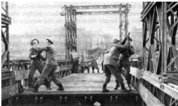
Class 70 Bascule Bailey Bridge being raised
